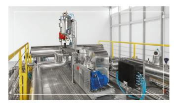
ATEX zone-1 rated, the gas room should be separated from the chamber room. We have a special design to allow the automatic changeover of the ETO containers, which are placed on weight scales.
